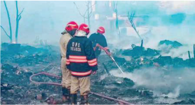
Firefighters at the site after a massive blaze destroyed huts in the Rithala area of Delhi on Thursday
