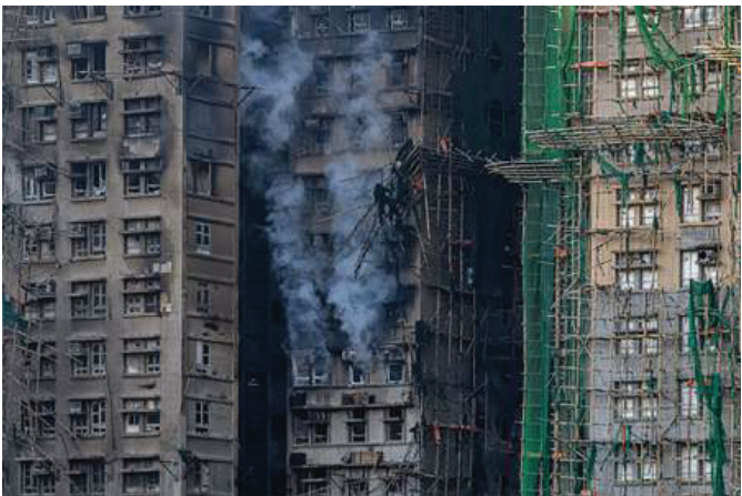
The charred high-rise after a deadly fire that started Wednesday at Wang Fuk Court, in Hong Kong
